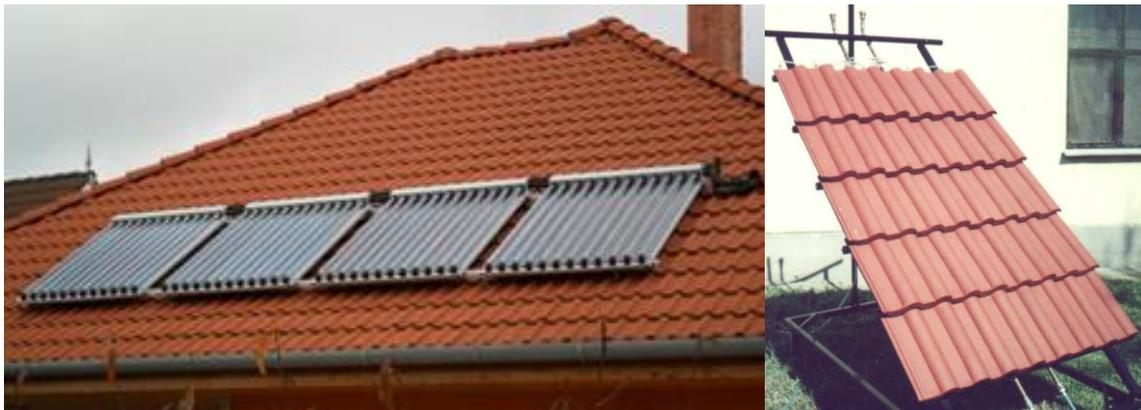
Fig. 1. The traditional and advanced structure design of solar collector
