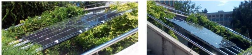
The system is divided into two subsystems, each of them partly covering the air wells in front of the building. Each subsystem is formed from 10 identical 165 W<sub>p</sub> modules, so the total nominal power of the system is 3,3 kW<sub>p</sub>.
